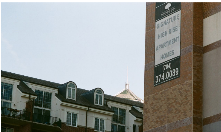
Figure 4: Signature High Rise Apartment Homes (Martin, 2022)
